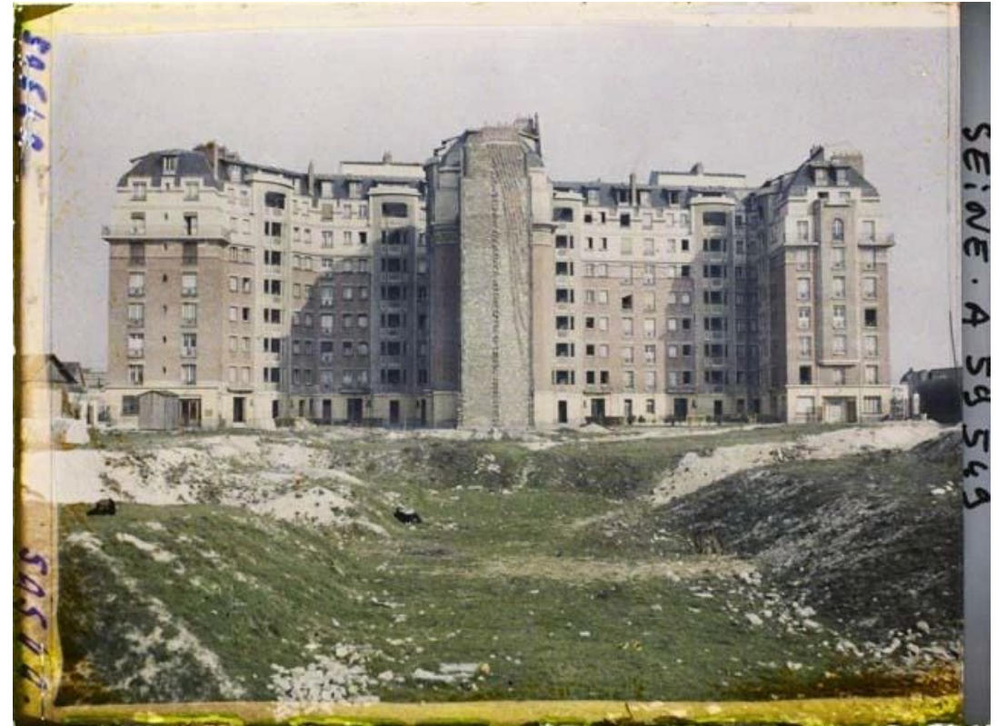
HBM "Art déco" on destroyed fortifications
